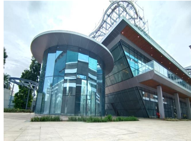
Mindspace Airoli East Highstreet (~0.05 msf) Completed (Part OC received)
