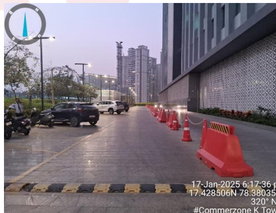
View of the Internal pathway
